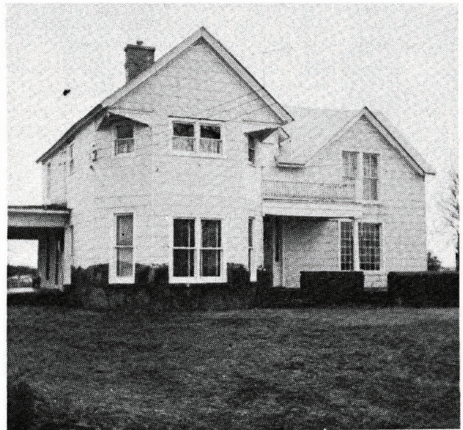
This is the House which will accommodate a maximum of ten children at FairHaven Children's Home.
